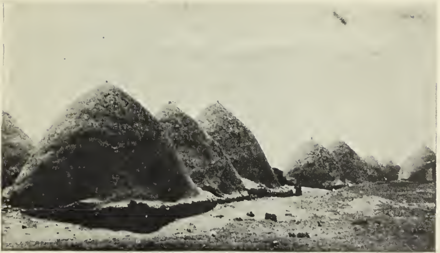
One of the "beehive" villages on the upper Euphrates. The windowless houses, which are built of sun-dried bricks, look like the noses of monster shells made for some titanic cannon.
